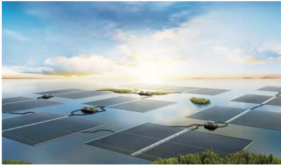
Lianghuai, Anhui 170MW floating project
