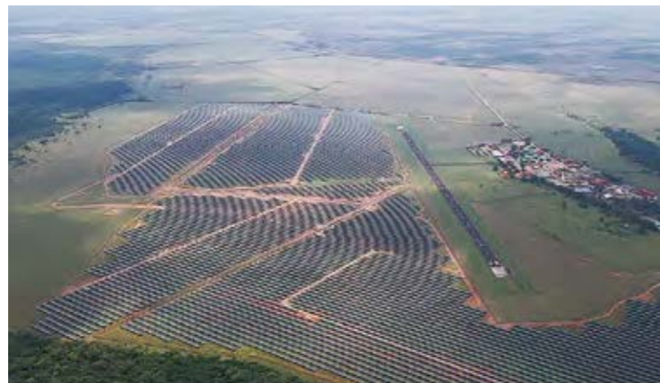
Los Llanos, Colombia 81.7 MW ground-mounted power station project
