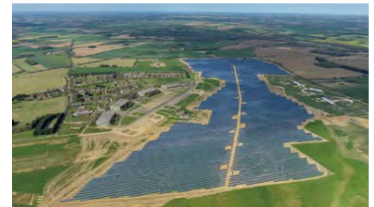
Norfolk, Britain 50MW ground-mounted power station project
